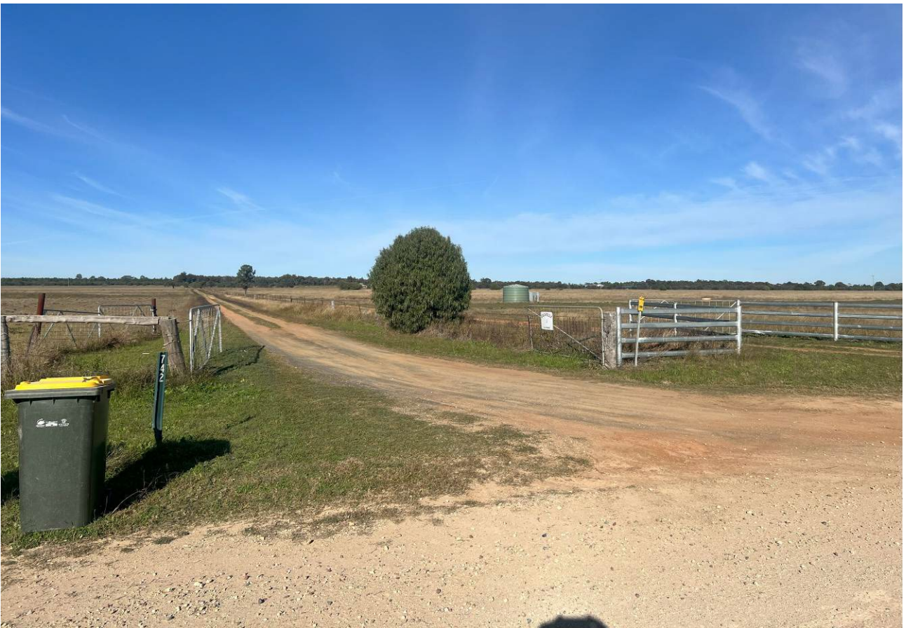
Photograph 2 – Existing site vehicular access and internal access road.
