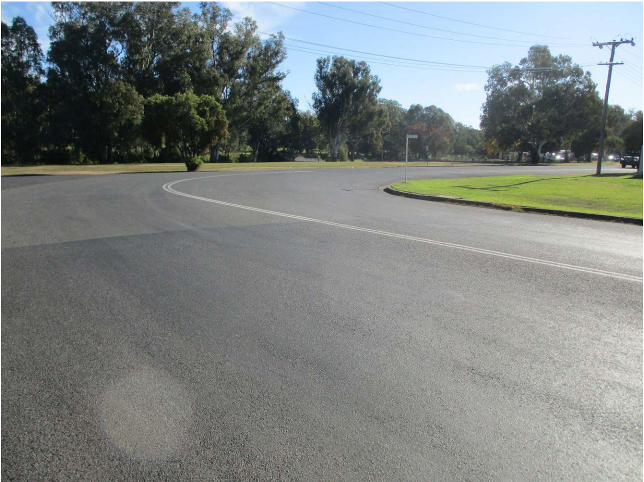
Photograph 4 – Tibbereena Street near Fitzroy Street.
